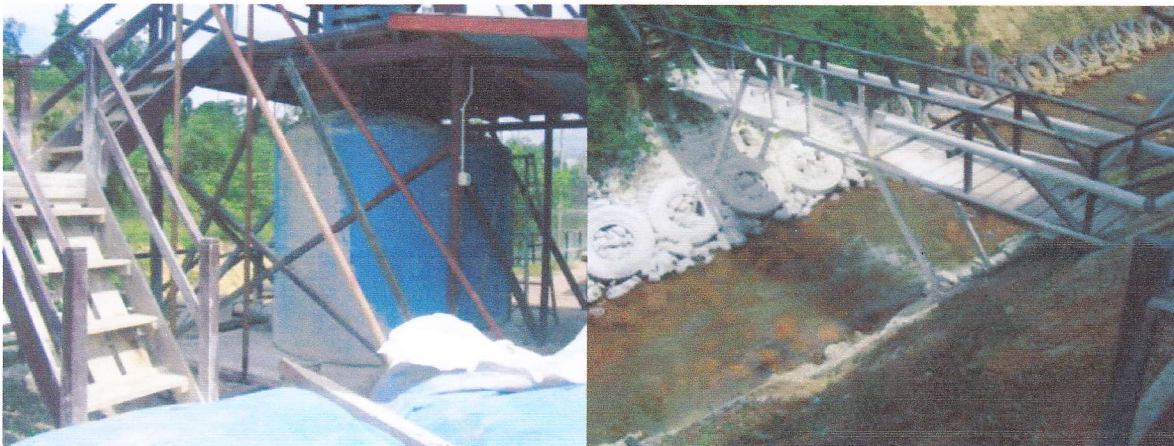
Fig. 4. Liming of AMD at PT. Kaltim Prima Coal
