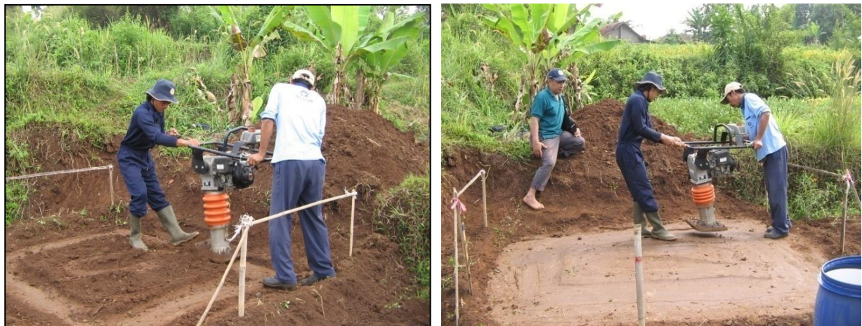
Figure 6. Construction of subgrade prototype
