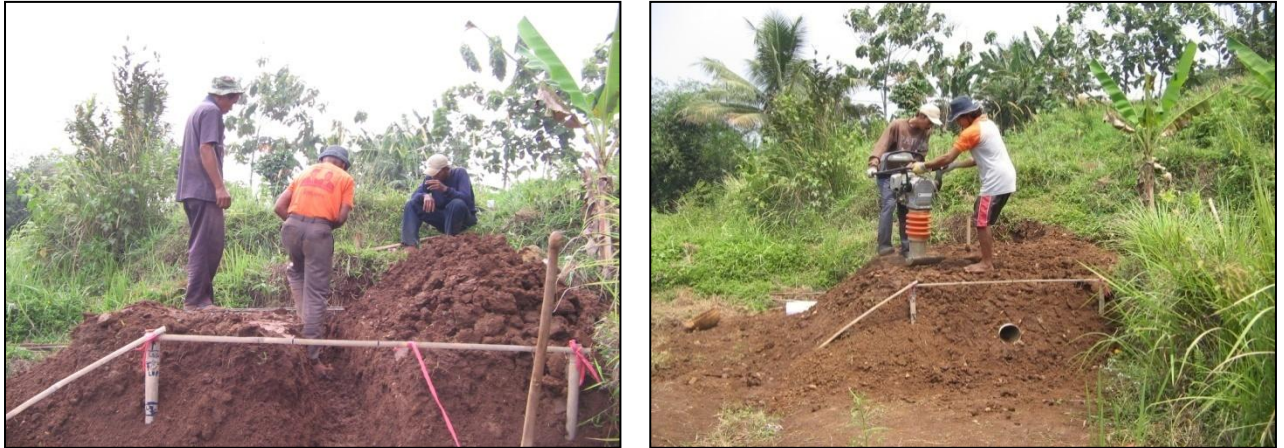
Figure 7. Irrigation pipeline installment
