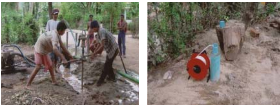
Figure 8. Bore-holes and measuring ground water level.
