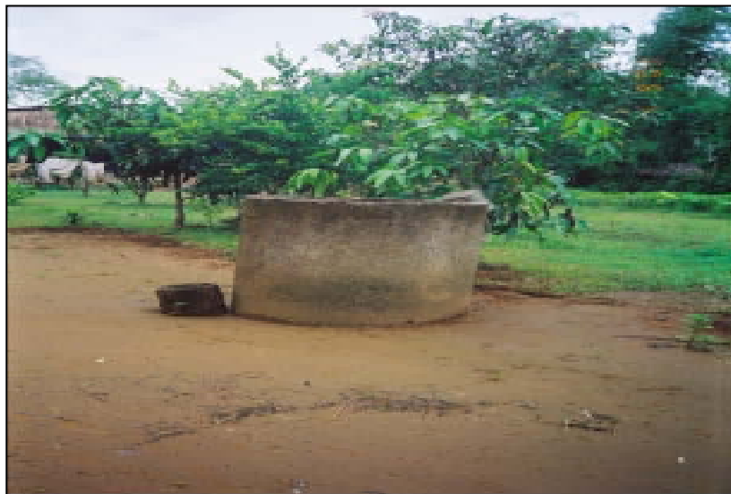
Figure 3. Cement- walled wells for domestic consumption and watering cashcrops in the study areas.
