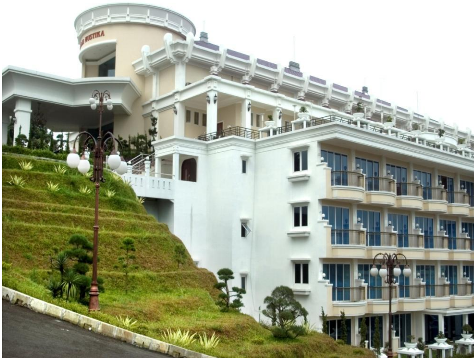
Braja Mustika Hotel & Convention Centre Building
