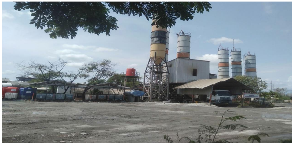
Gambar 46. Kondisi lapangan plant BSP Sayung
